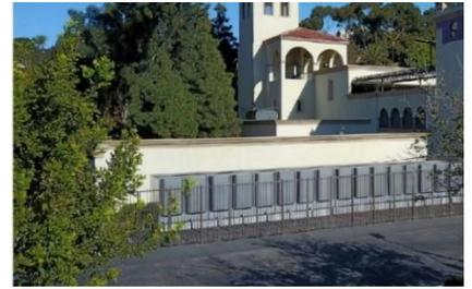
Bloom Energy has created Energy Server blocks that are repeatable and scalable. The most common base block for the global market is the 325 kW, as shown in Figure 1. With this 325 kW base block, the Energy Server is then duplicated and scaled to multiple megawatts to fit the needs of any project. There is no technical limit on the size of the Energy Server for primary power applications.
